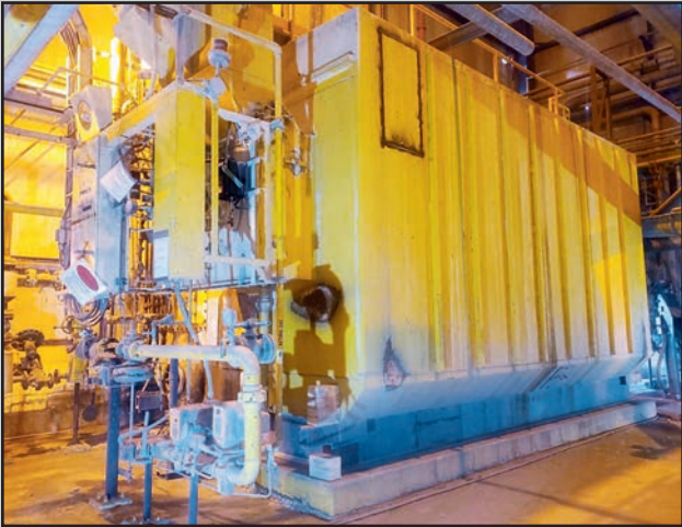
NEBRASKA PACKAGE STEAM BOILER
