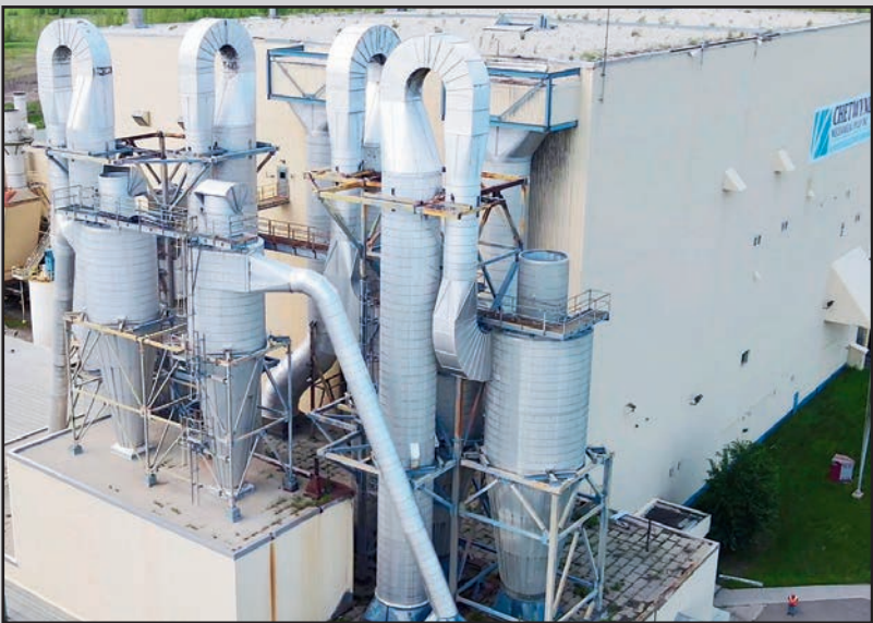
FLAKT DRYER DRYING CYCLONES
