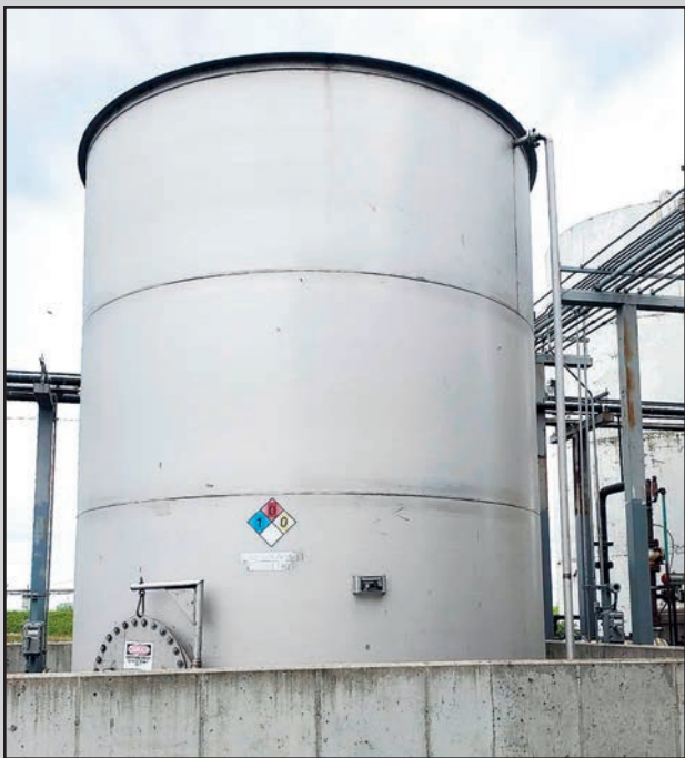
16,000-GALLON STAINLESS STEEL STORAGE TANK
