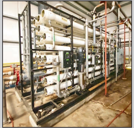
US WATERS 400 GPM RO SYSTEM
