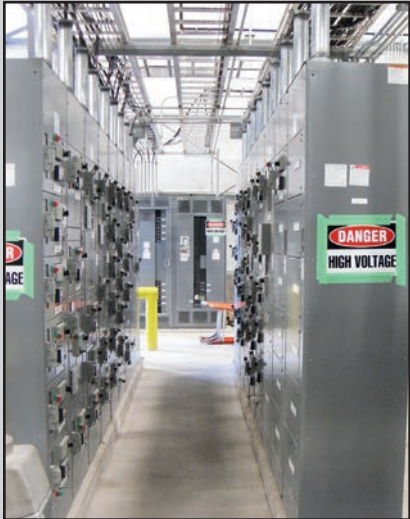
SQUARE D MOTOR CONTROL CENTERS
