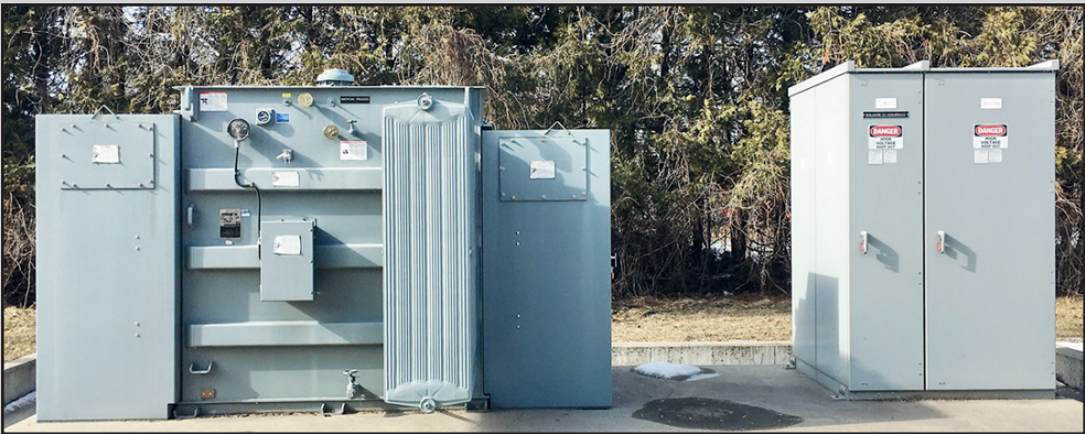
TRANSFORMER AND SWITCH GEAR
