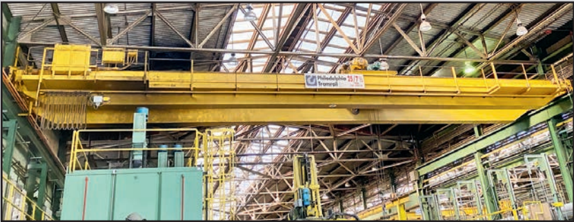
SAMPLE BRIDGE CRANE
