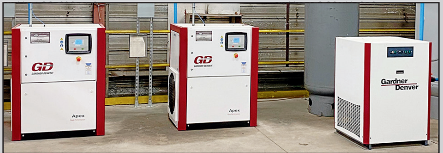
VIEW OF GARDNER DENVER AIR COMPRESSORS AND AIR DRYER
