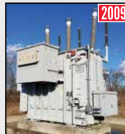
(14+) SIEMENS & VTC 169Kv/13.8Kv to 1,000-KVA Transformers
